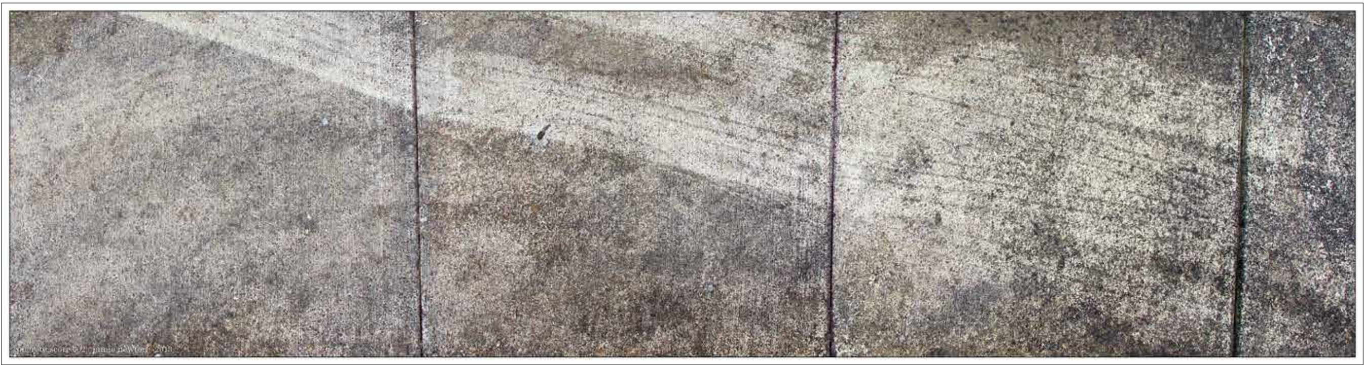
concrete score (002) • june 2013
